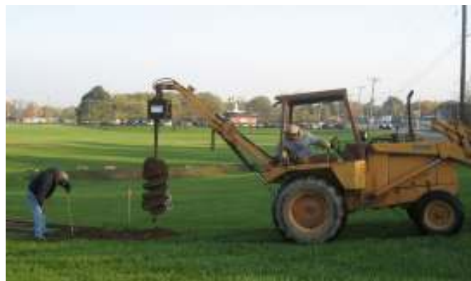
Drilling/digging holes for the Monument bases
